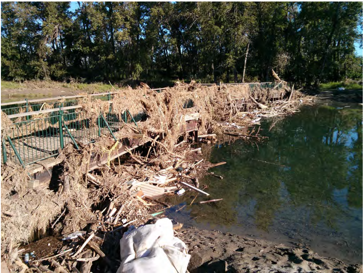
Aftermath of June 2013 Catastrophic Flooding
