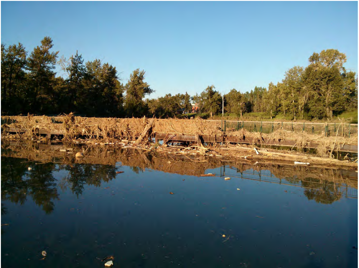
Aftermath of June 2013 Catastrophic Flooding
